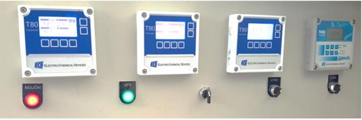
Sensors are connected to 4 smart instruments (two of them are holding two sensors each).
